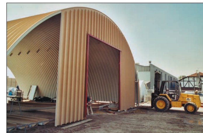
Door and window frames are installed as the end walls are being erected.
