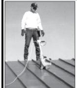
We have Powered Seamers available for lease for most roof systems and profiles
